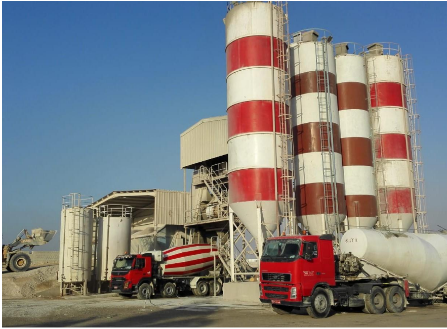
LIEBHERR Stationary Plant : Erected in 2008 Capacity 90m 3 /hr.
