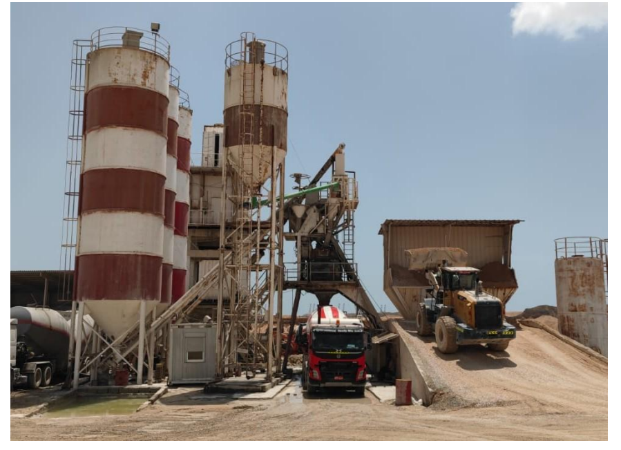
STETTER Semi Mobile Plant : Erected in 2013 Capacity 100m 3 /hr.
